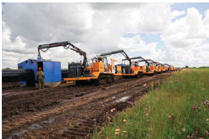
Figure 2. A full, large diameter welding spread.
